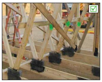
Install Web Member Permanent Lateral Restraint and Diagonal Bracing (or web reinforcement) and Bottom Chord Permanent Lateral Restraint and Diagonal Bracing as required. PHOTO B2-11
