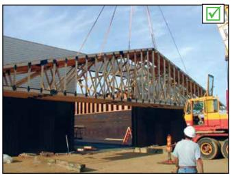
Pick up the finished assembly and set it into place. **PHOTO B2-12**
