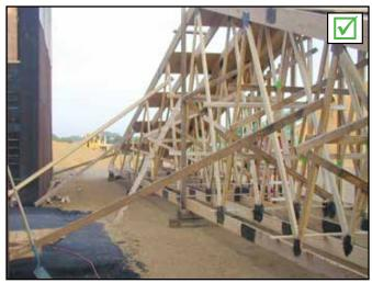
Ground Bracing for Truss assembly being built on the ground. **PHOTO B2-9**
