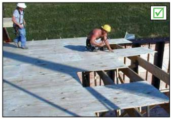
✓ Install All Permanent Individual Truss Member Restraint/ Bracing Immediately: Once the installation crew becomes familiar with the procedure, the Permanent Lateral Restraint and Diagonal Bracing for Webs and Bottom Chords can be installed in the time it takes to release the hoist and install the next Truss.
