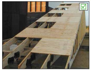
Install Structural Sheathing as soon as the first "set" of Trusses have been properly plumbed, restrained and braced. Begin at the heel and alternate 4'x8' and 4'x4' sheets up to the peak. **PHOTO B2-10**
