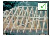
Proper bracing scheme - Continuous TCTLR with Diagonal Bracing. **PHOTO B2-7**
