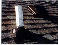
10. We will install two bath fan vents with an insulated duct. This will remove moist air from the attic, which can cause damage to the roof decking due to condensation. This is required to meet standard BUILDING CODE.
